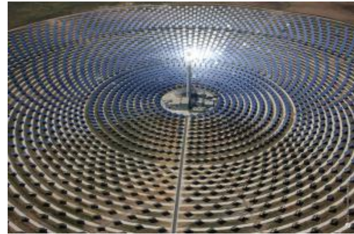
Solar power tower, Sevilla, Spain
