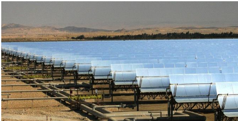
Parabolic trough, Egypt
